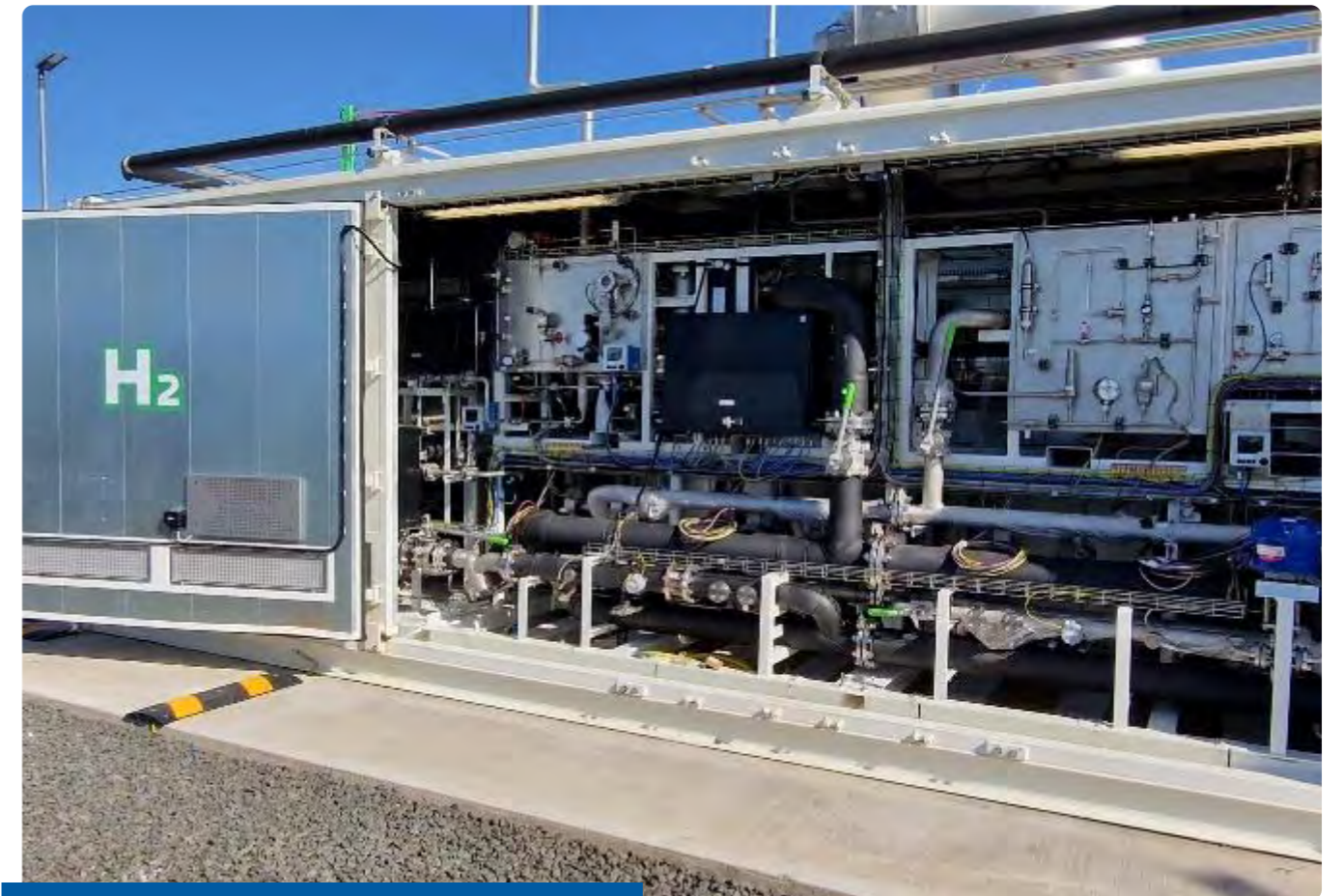
Electrolyser at our Long Mountain Wind Farm in Co. Antrim
